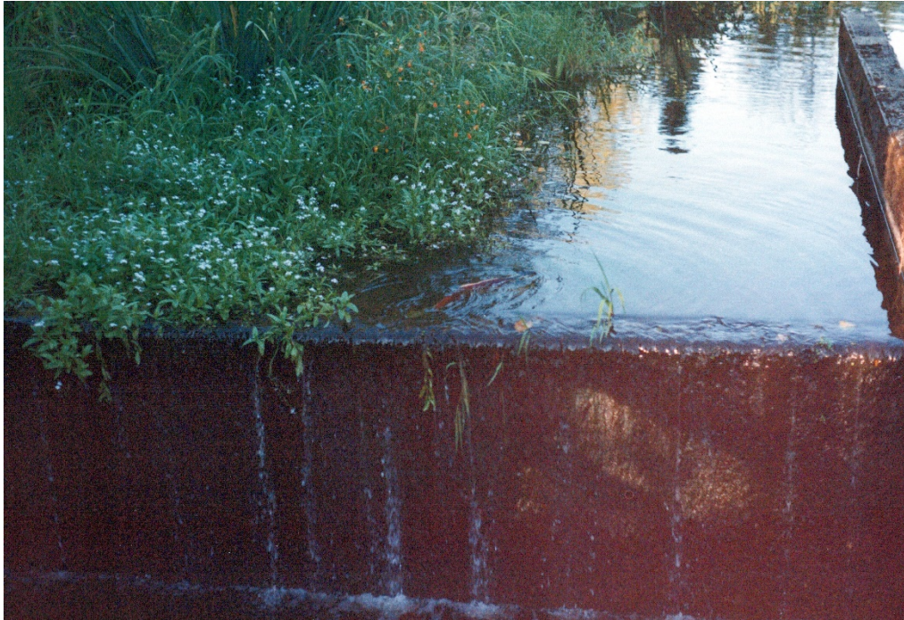
Figure 23. Water overflowing the dam and backwatering the channel upstream, October 1990.
