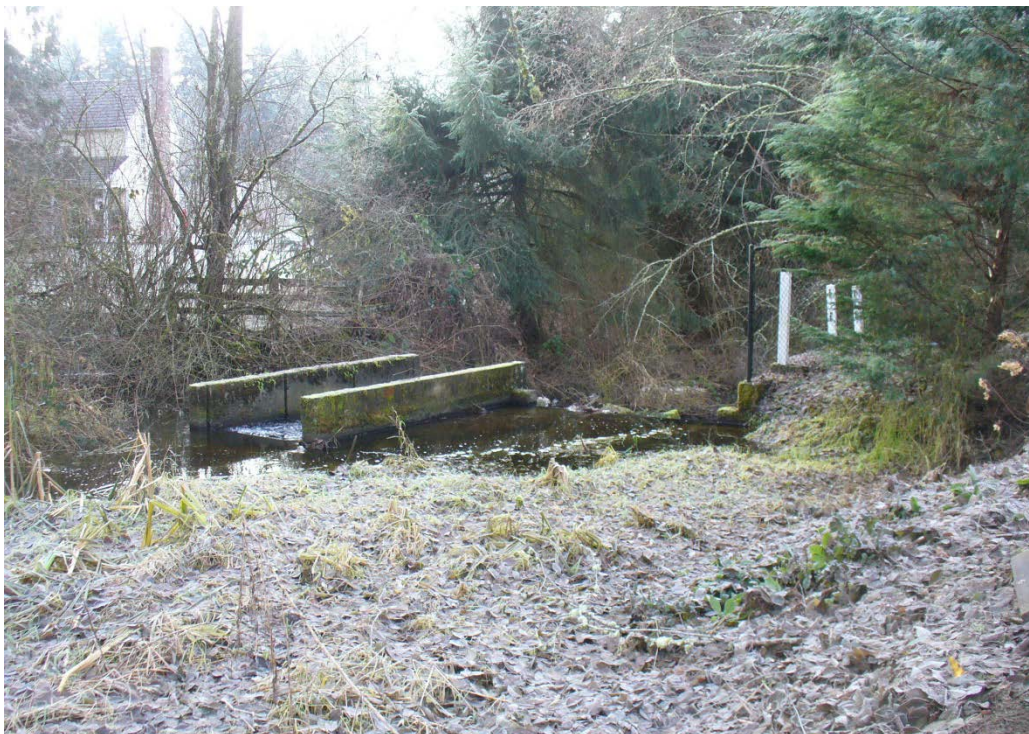
Figure 12. Facing southeast downstream from above the weir. Riverine wetland in foreground, fish ladder walls and weir in the center, a home in Homestead neighborhood is in the background, upper left. (1/17/23).
