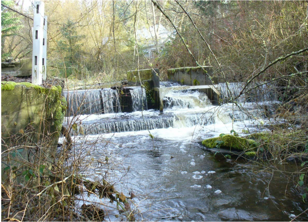
Figure 9. Existing weir and fish ladder (12/15/22).
